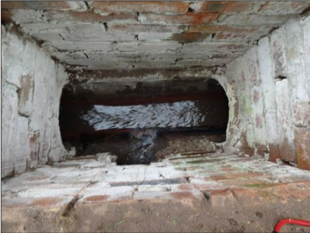
Photo: DSC02057.JPG 0m, Start node type, manhole, reference number : 01
