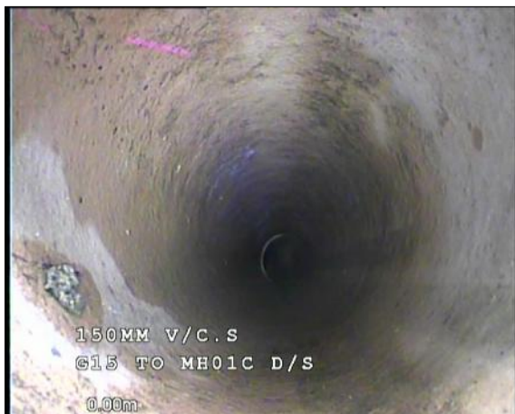
Photo: 23_23_263_A.jpg, 00:00:06 0m, Water level, 05% of the vertical dimension
