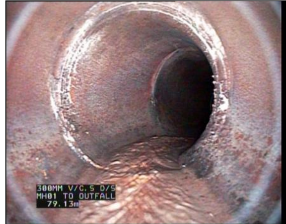
Photo: 12_12_144_A.jpg, 00:12:32 79m, Line deviates right
