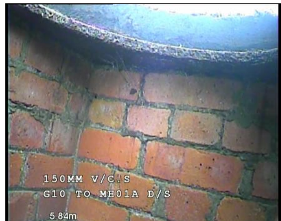
Photo: 10_10_100_A.jpg, 00:01:09 5.8m, Finish node type, manhole reference number: 01A
