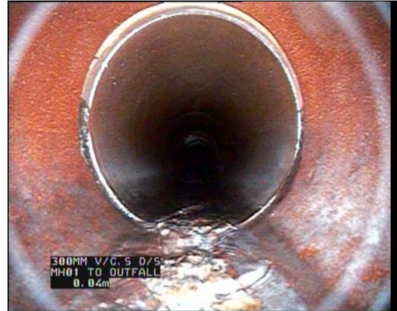
Photo: 12_12_28_A.jpg 0m, Water level, 10% of the vertical dimension Remarks: HEAVY FOUL POLLUTION THROUGHTOUT
