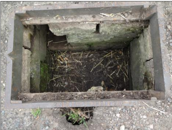
Photo: DSC02159.JPG 0m, Start node type, gully, reference number : G02A Remarks: GULLY 02A
