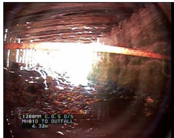
Photo: 27_27_299_A.jpg, 00:00:50 4.3m, Finish node type, outfall reference number: OUTFALL
