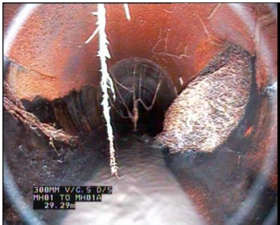
Photo: 13_13_169_A.jpg, 00:04:41 29.3m, Roots, mass, 10% cross-sectional area loss Remarks: POSSIBLE REDUNDANT CONNECTION
