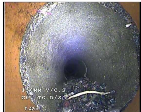
Photo: 7_7_75_A.jpg, 00:00:14 0.5m, Material changes, concrete
