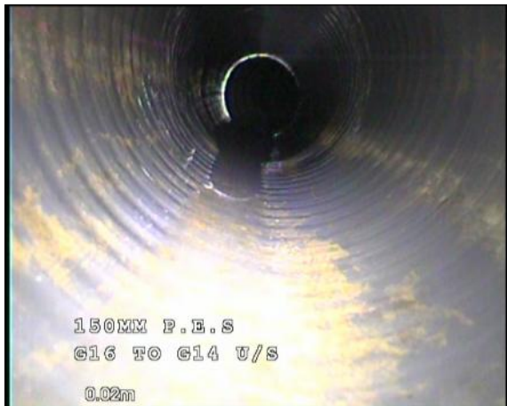
Photo: 17_17_226_A.jpg, 00:00:06 0m, Water level, 05% of the vertical dimension
