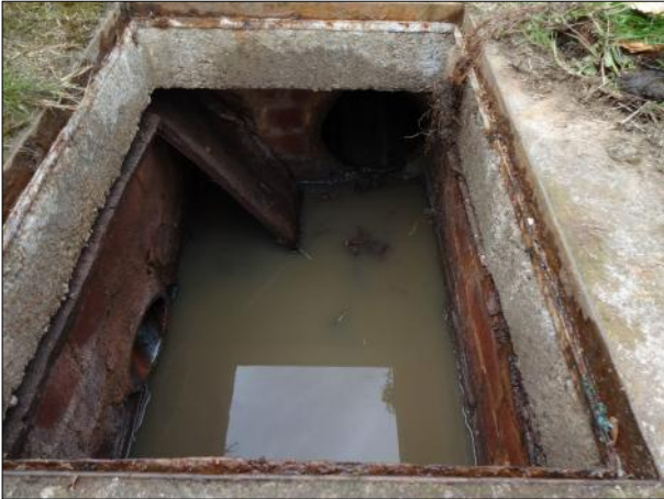
Photo: DSC02164.JPG 0m, Start node type, manhole, reference number : 01F
