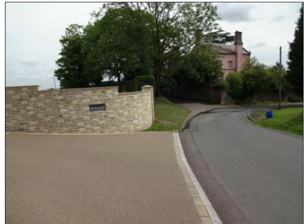
Photo: DSC02167.JPG, 00:00:58 1.3m, General photograph taken at this point Remarks: SURFACE WATER RUNNING FROM PRIVATE DRIVE. ASSUMED COLLAPSED PIPE AHEAD
