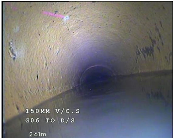
Photo: 6_6_69_A.jpg, 00:00:43 2.6m, Water level, 75% of the vertical dimension
