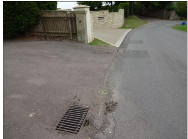
Photo: DSC02161.JPG, 00:00:14 0m, General photograph taken at this point Remarks: LOCATION PHOTO
