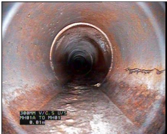
Photo: 11_11_23_A.jpg 0m, Water level, 10% of the vertical dimension Remarks: HEAVY FOUL POLLUTION THROUGHOUT
