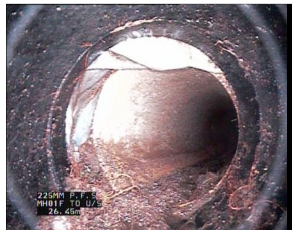
Photo: 32_32_352_A.jpg, 00:04:22 26.4m, Line deviates right
