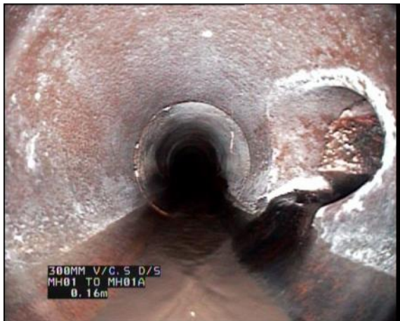
Photo: 13_13_30_A.jpg 0m, Water level, 10% of the vertical dimension Remarks: HEAVY FOUL POLLUTION THROUGHOUT
