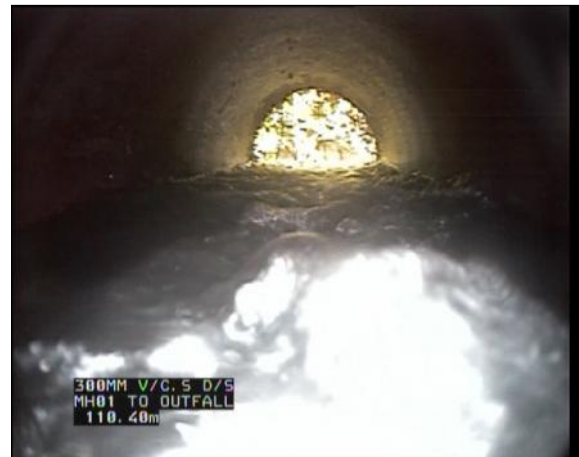
Photo: 12_12_152_A.jpg, 00:22:16 111m, Finish node type, outfall reference number: OUTFALL
