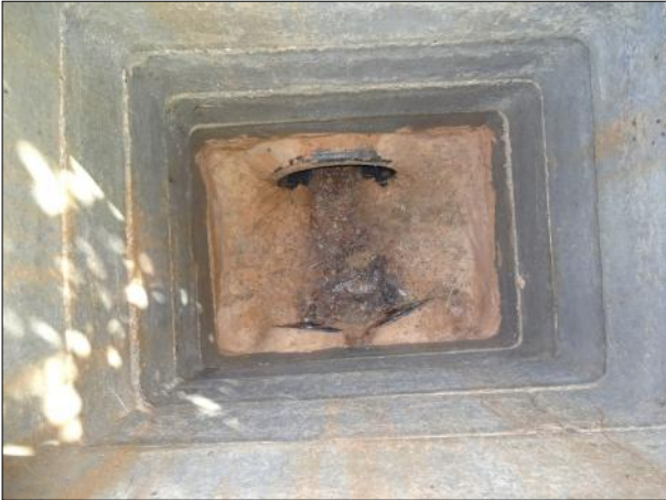
Photo: DSC02074.JPG 0m, Start node type, manhole, reference number : 01B
