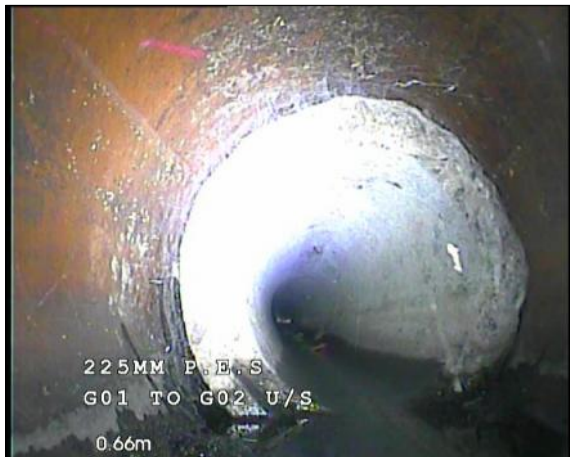
Photo: 3_3_38_A.jpg, 00:00:23 0.7m, Dimension changes, 150mm high Remarks: POOR REDUCER
