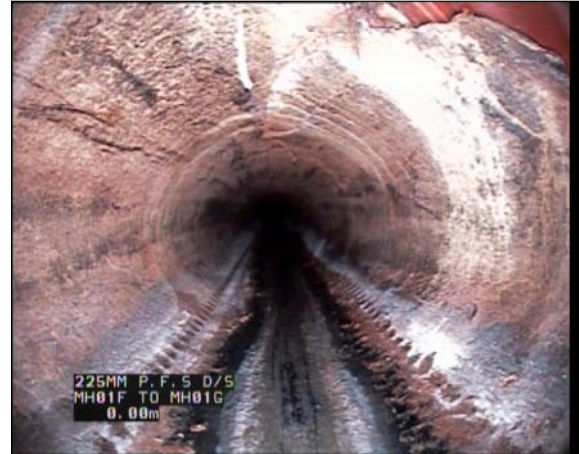
Photo: 1_1_10_A.jpg, 00:00:06 0m, Attached deposits, grease, from 7 to 5 o'clock, 5% cross-sectional area loss Remarks: HEAVY FOUL POLLUTION THROUGHOUT
