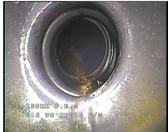
Photo: 19_19_233_A.jpg, 00:00:06 0m, Water level, 05% of the vertical dimension
