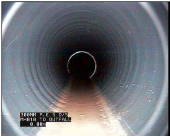
Photo: 25_25_276_A.jpg, 00:00:04 0m, Water level, 10% of the vertical dimension
