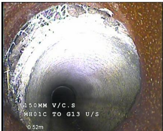
Photo: 24_24_275_A.jpg, 00:00:19 0.5m, Survey abandoned Remarks: OVERLAP COMPLETE TO POOR JOINT
