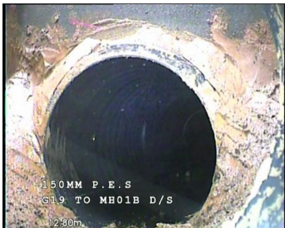
Photo: 21_21_242_A.jpg, 00:01:55 12.8m, Finish node type, manhole reference number: 01B
