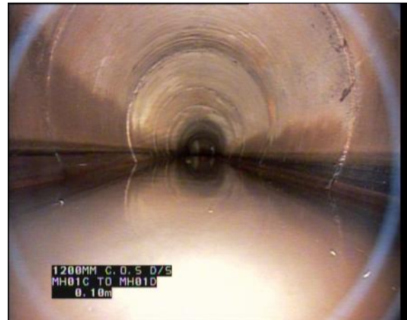
Photo: 26_26_286_A.jpg, 00:00:08 0m, Water level, 25% of the vertical dimension
