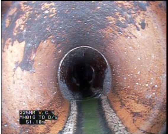
Photo: 33_33_392_A.jpg, 00:11:39 51m, Survey abandoned Remarks: UNABLE TO CONTINUE DUE TO TRACTION/GREASE
